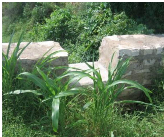
Water drainage system to drain rain water and reduce erosive force
